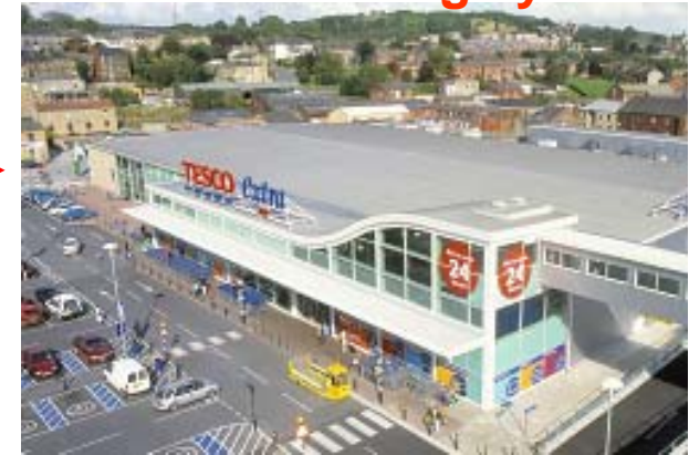
District heating system
