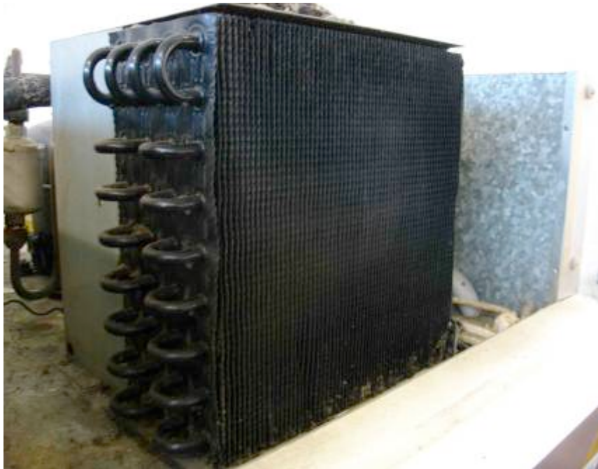
Figure 3. Top mounted condenser unit after cleaning
