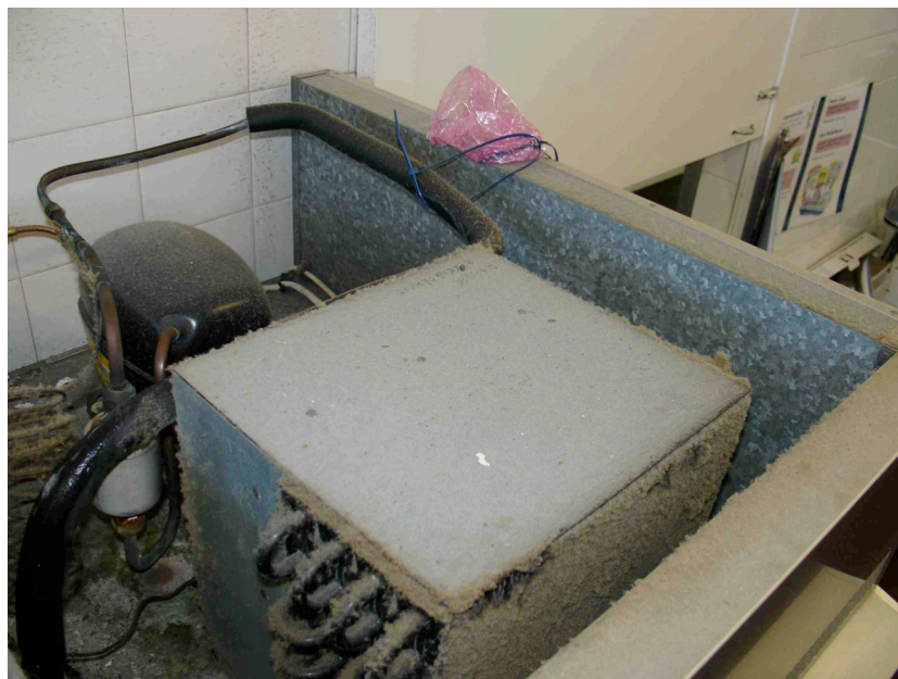
Figure 2. Top mounted condenser unit prior to cleaning
