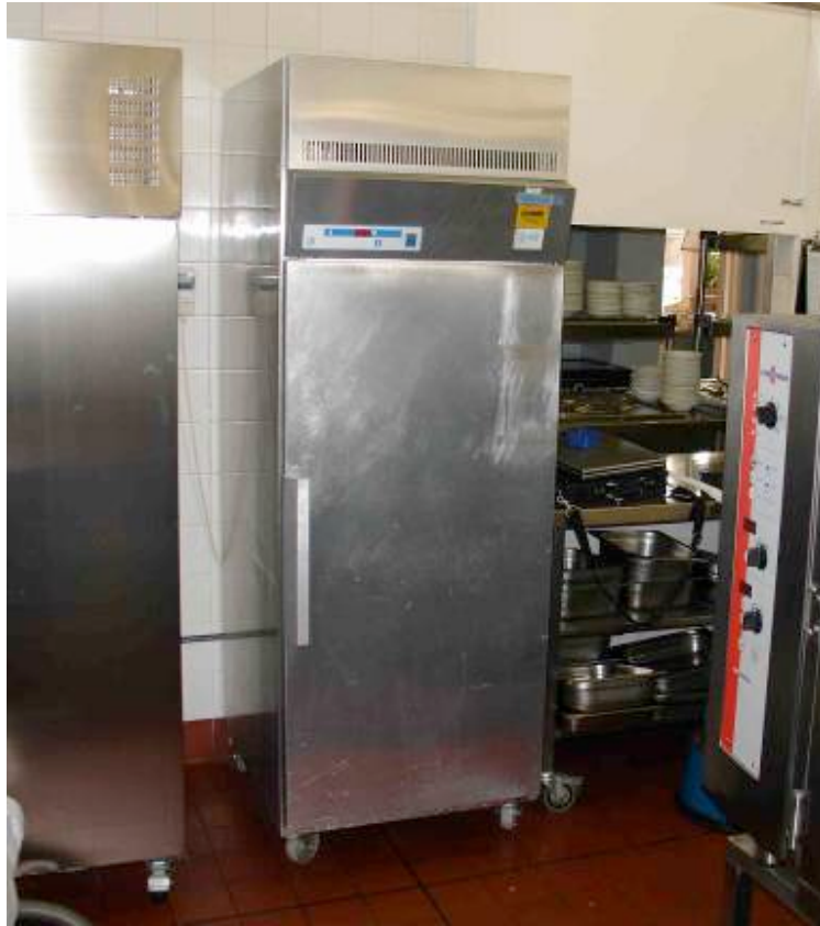
Figure 1. Upright commercial service cabinet freezer in canteen
