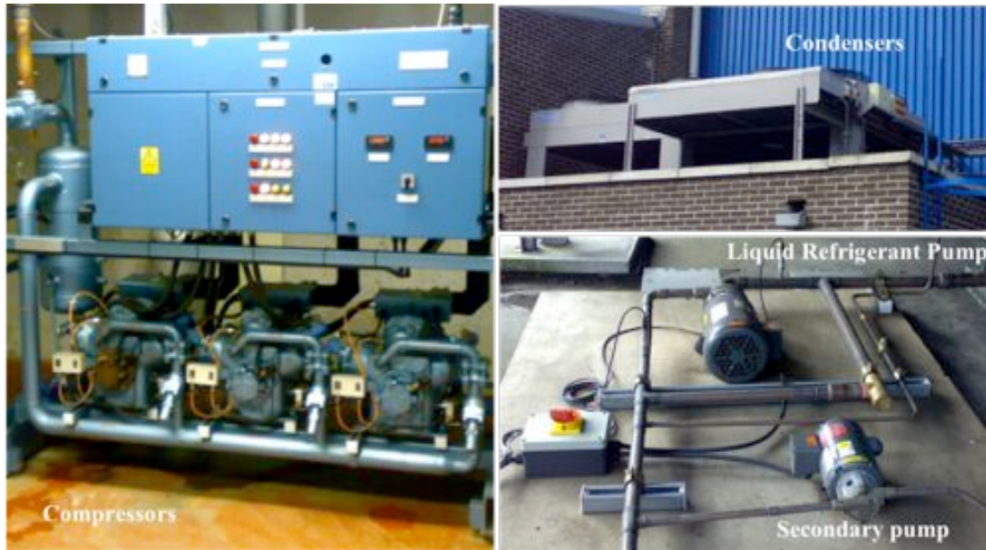
Figure 2: Refrigeration System Components
