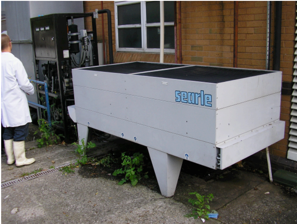
Figure 5. External housing of multi-compressor pack (black frame) and horizontal condenser fan unit (foreground)
