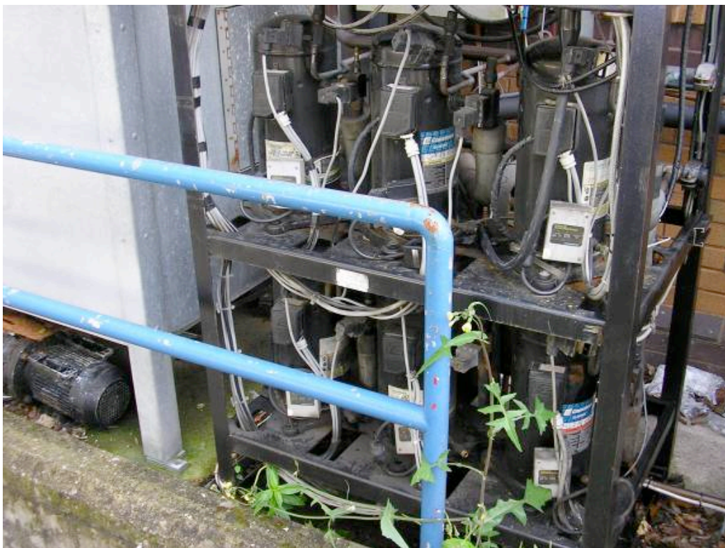
Figure 6. View of the multiple scroll compressor pack (3 above, 3 below)
