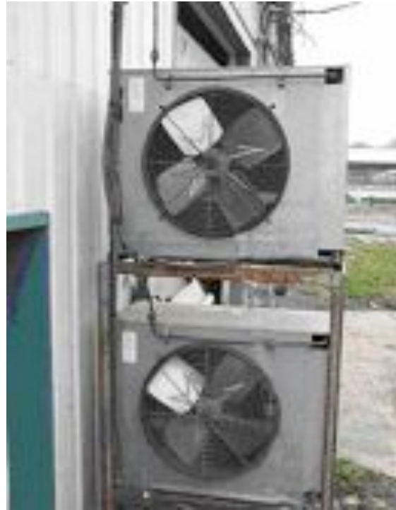
Example of a remote air-cooled condenser on dairy farm
