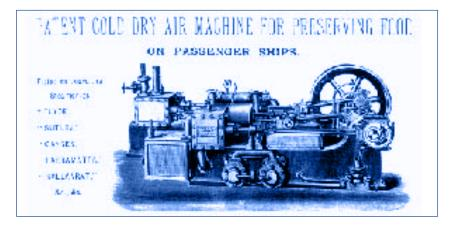
Air cycle is not a new technology. Air cycle or 'cold air machines' were available from companies such as J & E Hall (see picture) in the early 1900s. These were used on board ships and by food producers and retailers to provide cooling for their food stores.
